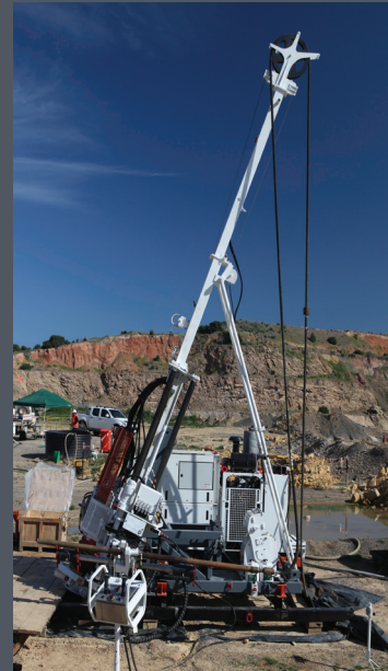
Surface Coring Rigs
